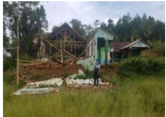
School damage totally in Bantarsari
